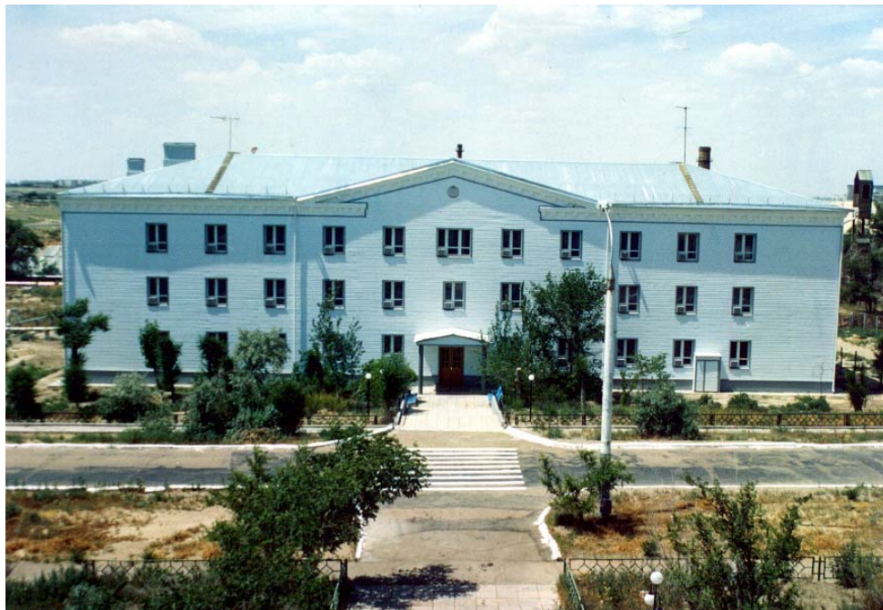
Figure 6-16. Hotel 1 at Site 2Zh Near the Site 254 PPF
